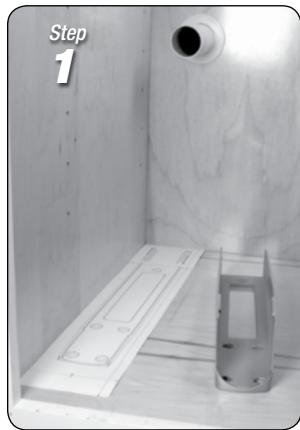
Use template provided to determine mounting base location. Read instructions on template for position. Side clearance will vary depending on cabinet. Tape template down to be more secure during marking or pre-drilling.
