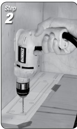
Once the location is confirmed, pre-drill or mark the 5 holes shown with an X on the template. Use a 5/64" drill bit to eliminate splitting or cracking in the wood.
