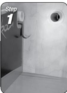
Dry fit your assembly with the escutcheon plate (*label side in hole*) and wire in place (*the escutcheon plate is notched for the wire to run through it along side the tubing*). Use a combination of short/long 90° or 45° fittings. Glue and assemble your fittings/tubing and attach to the trunk line. Do not glue the vacuum line to the fitting on the Vroom. Attach the low voltage wires from the Vroom to the low voltage wires coming from the trunk line using wire nuts.
