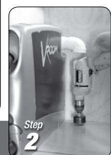
Using a hole saw bore a 2 1/4" hole through the cabinet and the floor.
